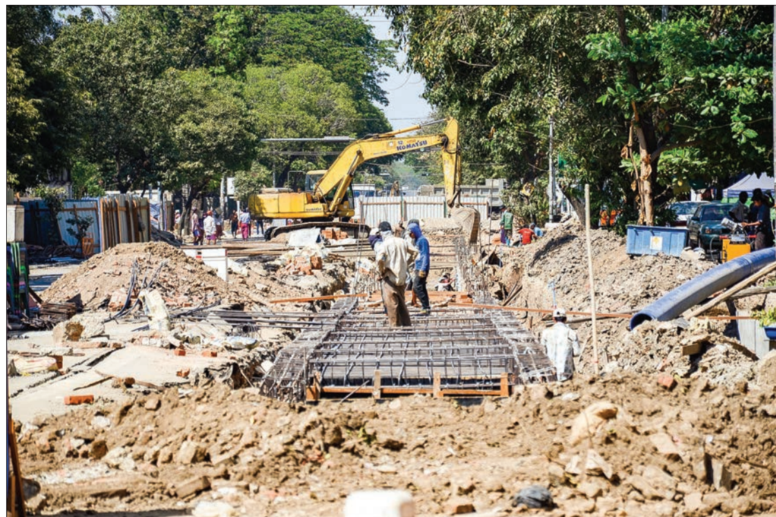
Workers seen at the upgrading of drainage system in Yangon. PHOTO: PHOE KHWAR
