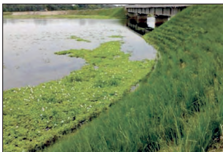
Growing vetiver as retaining wall along dam
