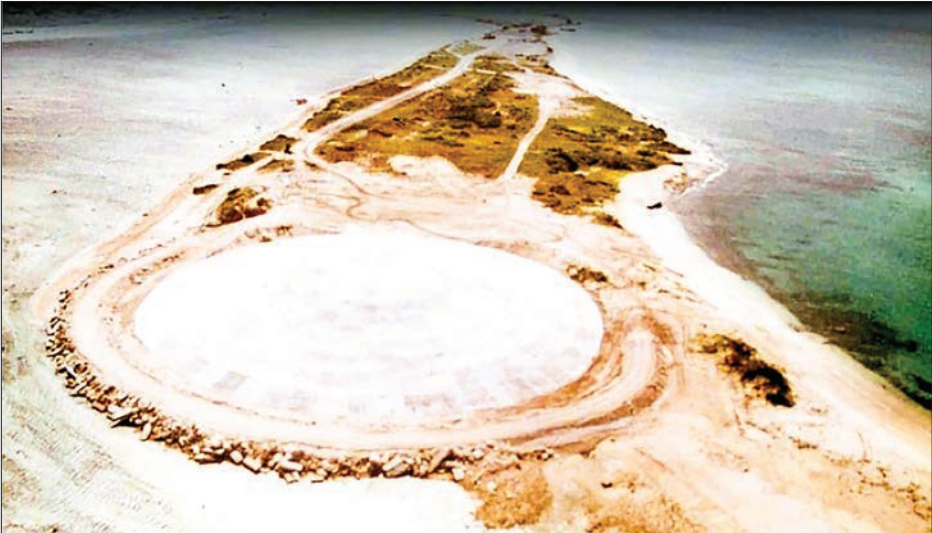
The huge dome built over top of a crater left by one of the nuclear tests over Runit Island in Enewetak in the Marshall Islands. PHOTO: AFP
