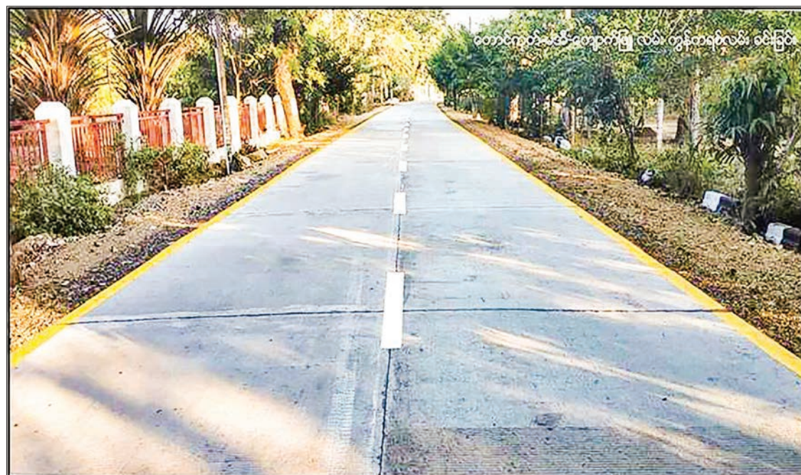
Newly built Taungup-Maei-Kyaukphyu concrete road. PHOTO:MNA
