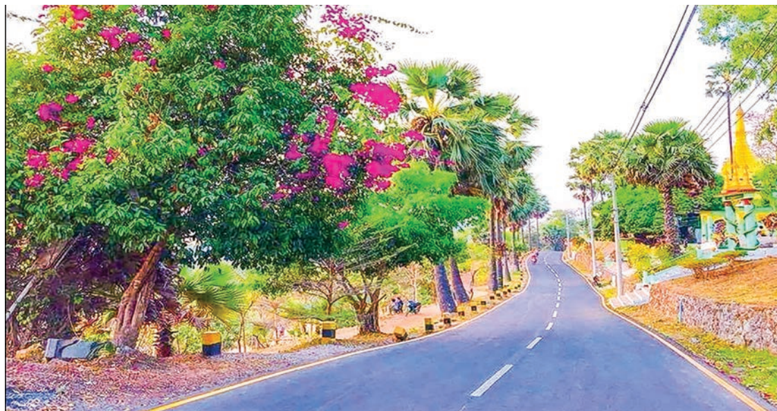
Taung Yoetan asphalt road constructed in Mawlamyaing Township.
