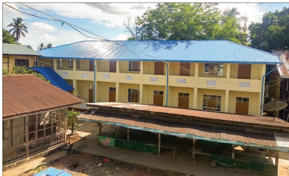
New school buildings are under construction in Mon State.
