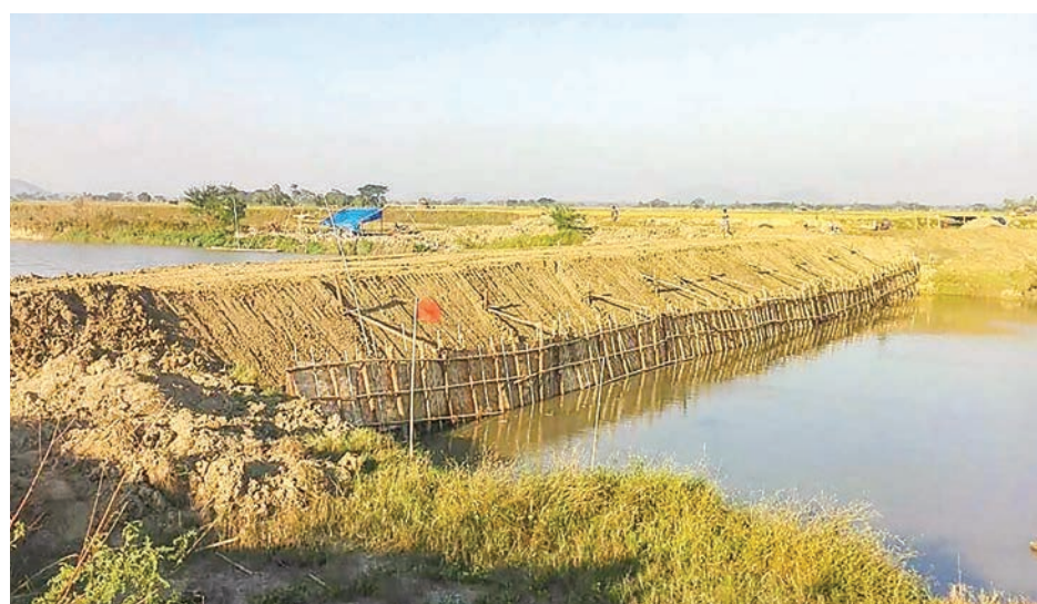
An embankment seen for water control system during summer paddy cultivation in Mon State.
