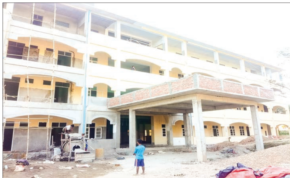
Extended building being constructed for Mawlamyaing General Hospital under construction.
