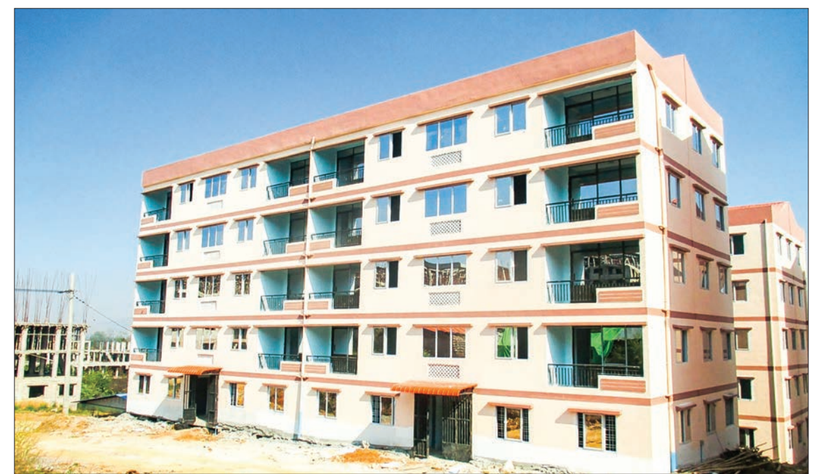
Low-cost housing for public provided within three year period in Shan State. PHOTO: MNA
