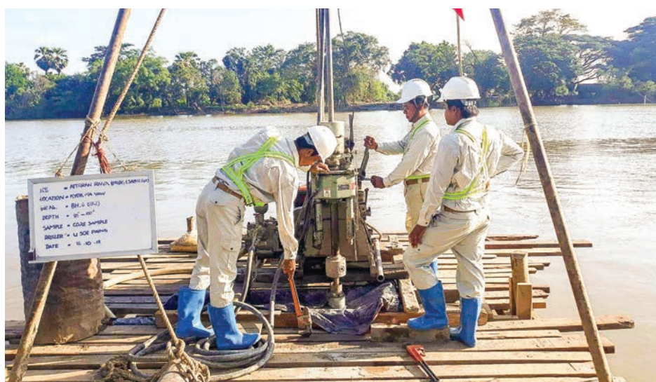
Engineers test soil samples for building the bridge across the Ahttayan River in Mon State.
