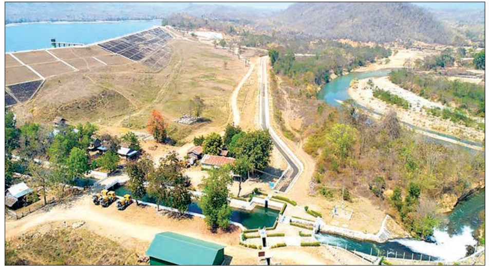
Rock lining underway along the embankment wall of Mahn reservoir in PinU Village, Ngaphe Township.
