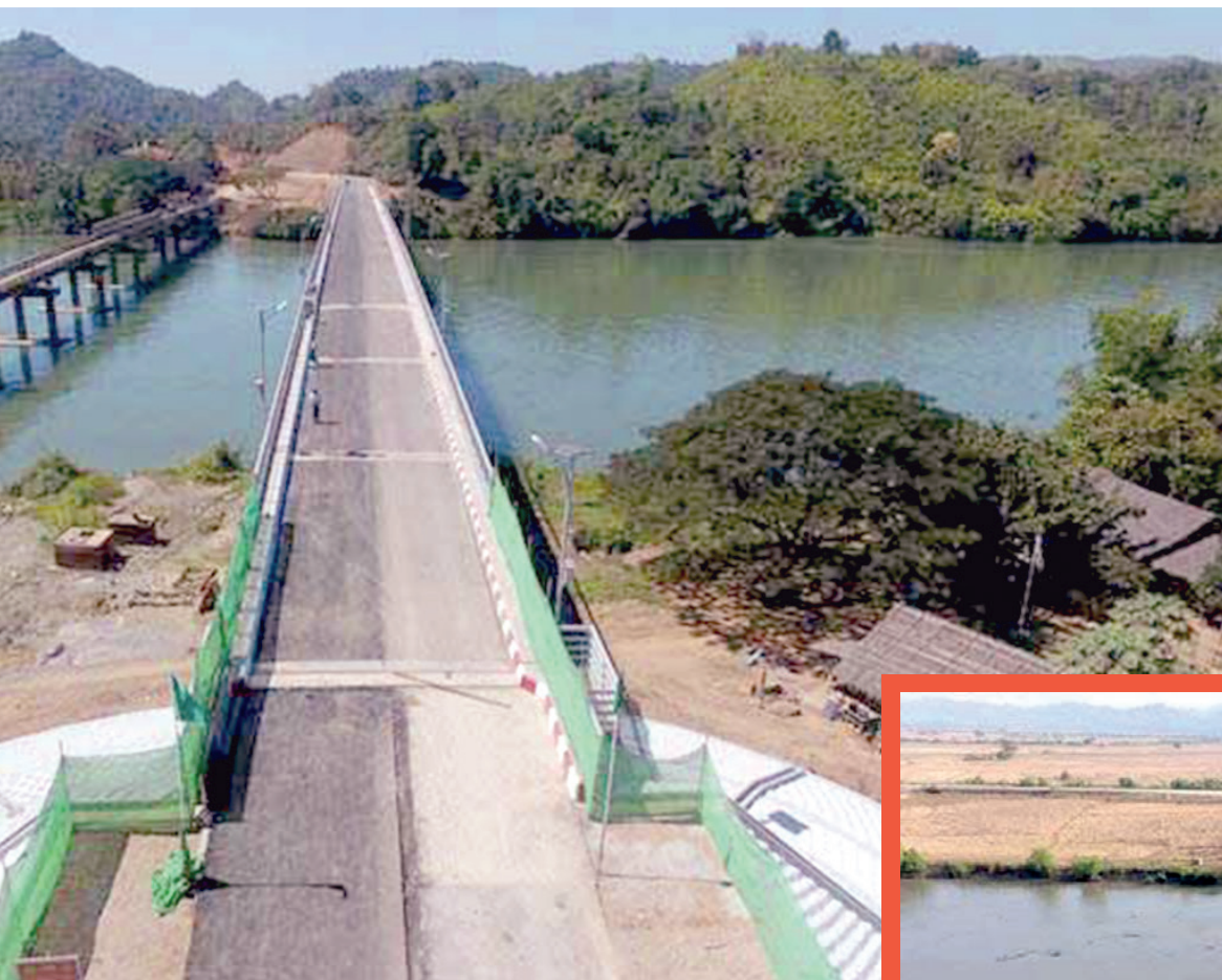
Darlet Creek Bridge. PHOTO: TIN TUN (IPRD)
