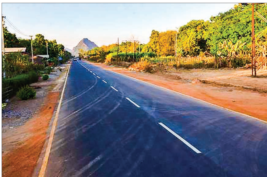
The Eindu-Zarthabyin road expanded and paved with nylon concrete.
