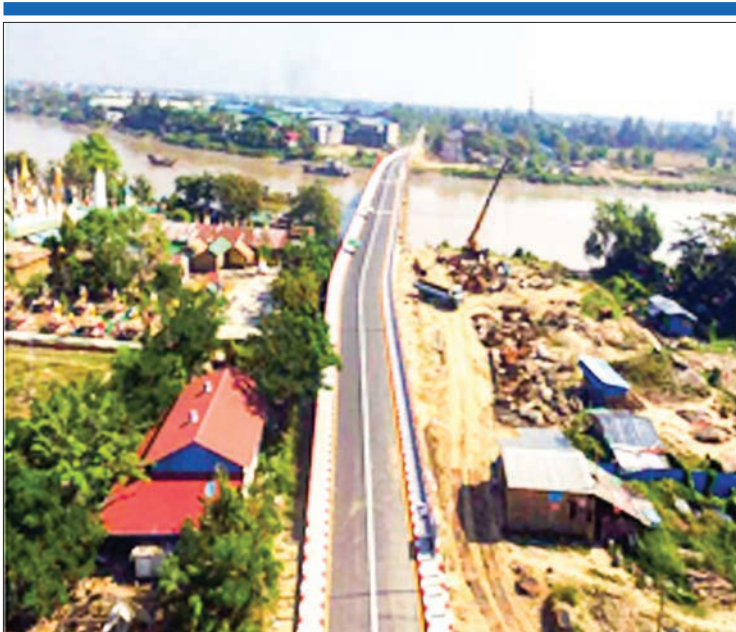
Photo shows a bridge which is under construction in Yangon.
