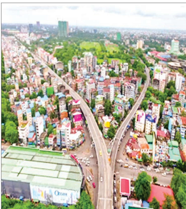
Bird's eye view of the construction of Hledan flyover in Yangon.
