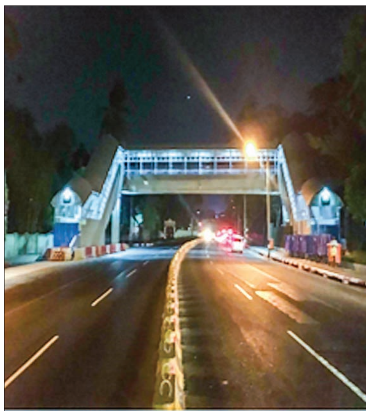
Photo shows the under-construction flyover at Myaynigone in Yangon.
