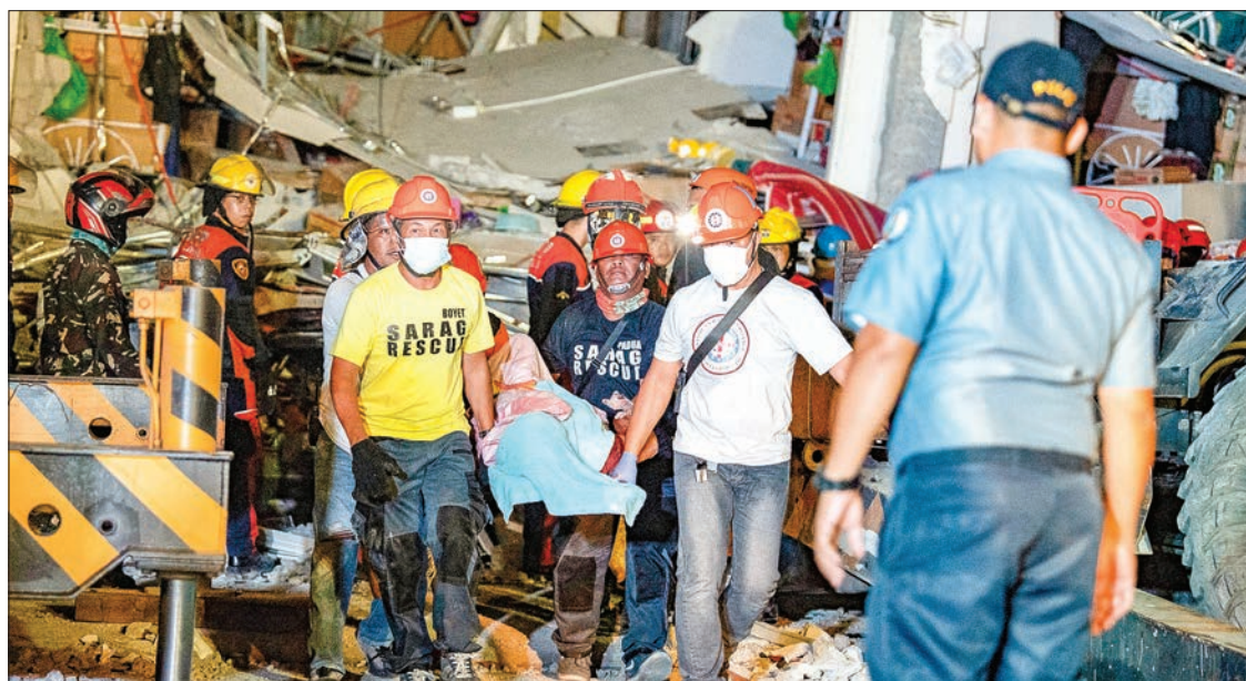
Rescue workers carry victim from a collapsed Chuzon Super Market in Porac, Pampanga, after a powerful earthquake hit northern Philippines on 22 April 2019. At least five people were killed when buildings collapsed near Manila after a powerful earthquake set skyscrapers swaying and drove terrified locals into the street. PHOTO: AFP
