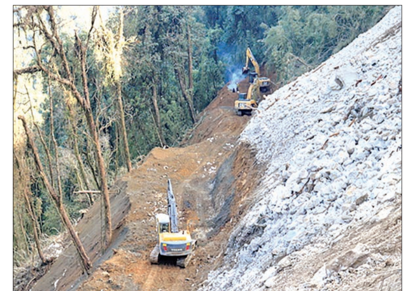
Machines paving into the Maggwayza-Khaunglanphu road section.
