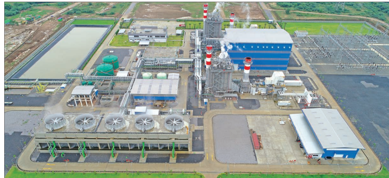
225MW Mingyan power plant
