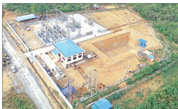
66kV Pathein-Ngwe Saung Transmission Line & Substation
