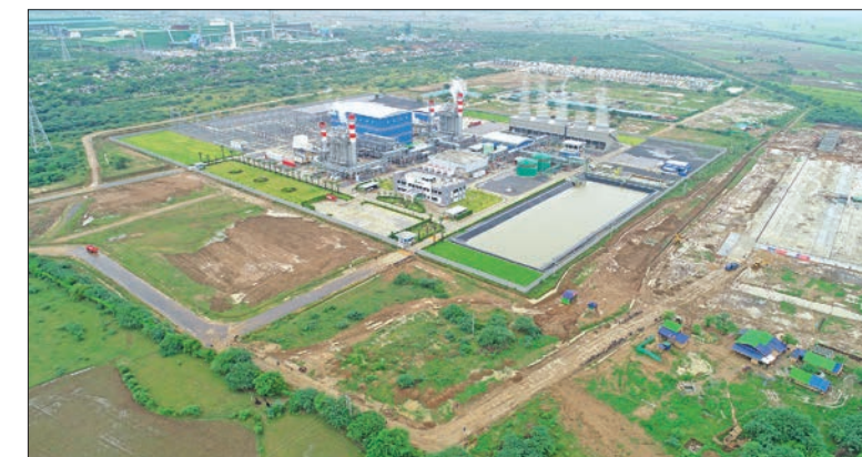
225MW Mingyan power plant
