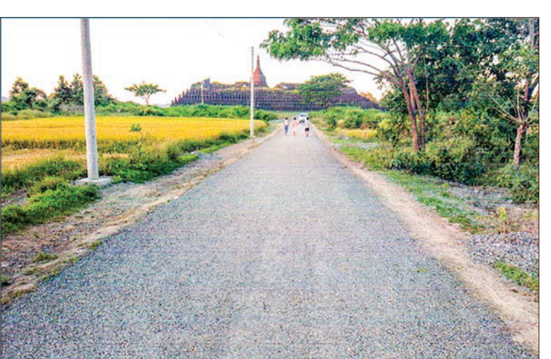
Photo shows the completion of Kothaung Phayar Road construction in MraukU Township, Rakhine State. PHOTO: MNA
