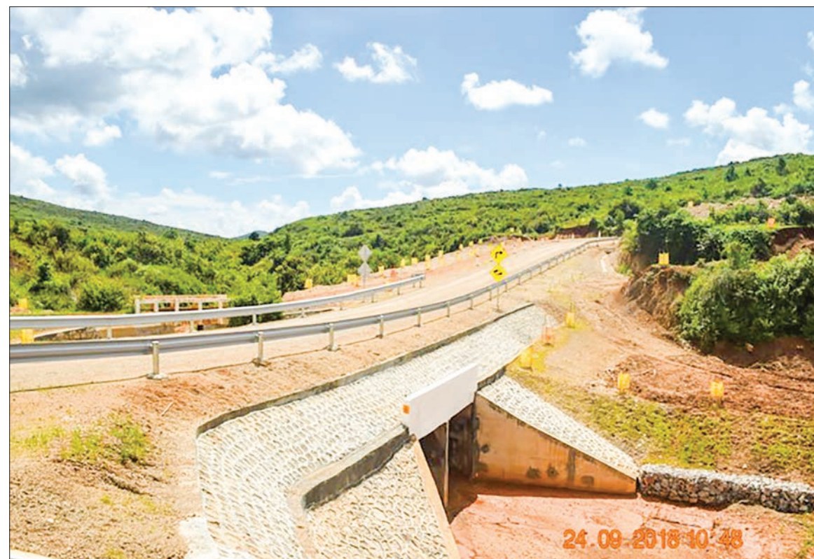
Photo shows the completion of Bawmin-Hsupaninn-Kanparni-Thayetpu road construction under the rural development programme provided by German Development Bank. PHOTO: MNA
