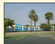
Renovation of Sittwe General Hospital
