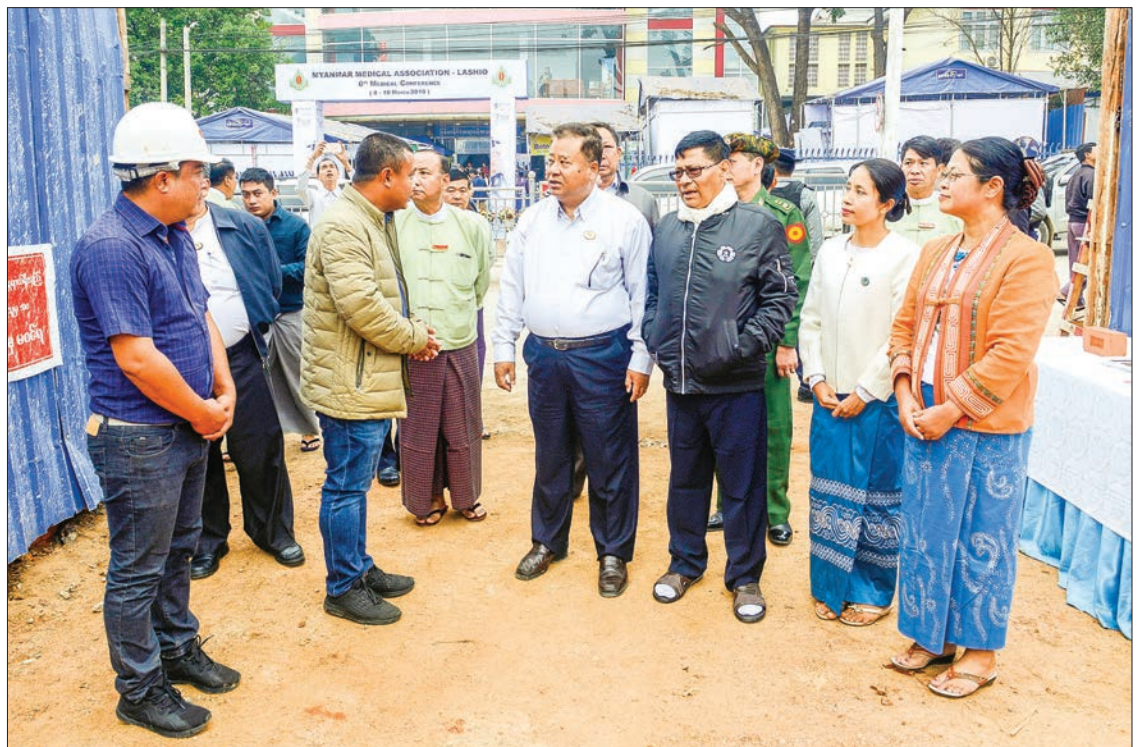
Chief Minister Dr. Lin Htut inspects ongoing construction of the 7-storey RC building for the community centre in Lashio yesterday. PHOTO: HAN LIN (LASHIO), DISTRICT IPRD
