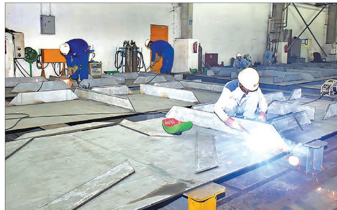
Workers welding steel frames at the J&M Steel factory.
