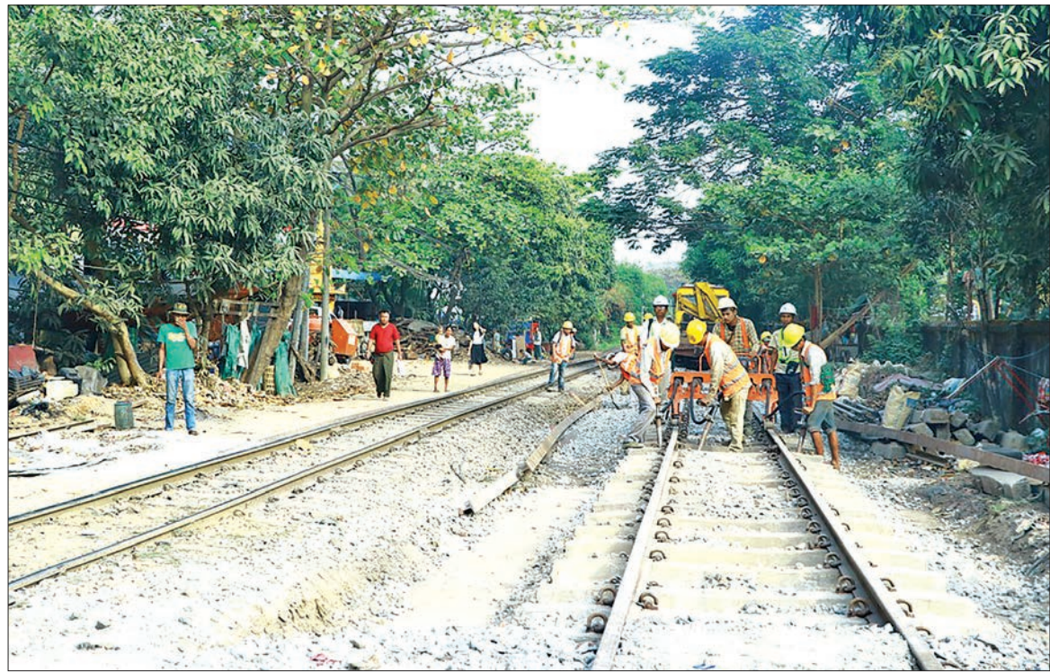
Track upgrading work underway to improve Yangon Circular Trains Service. PHOTO: MNA
