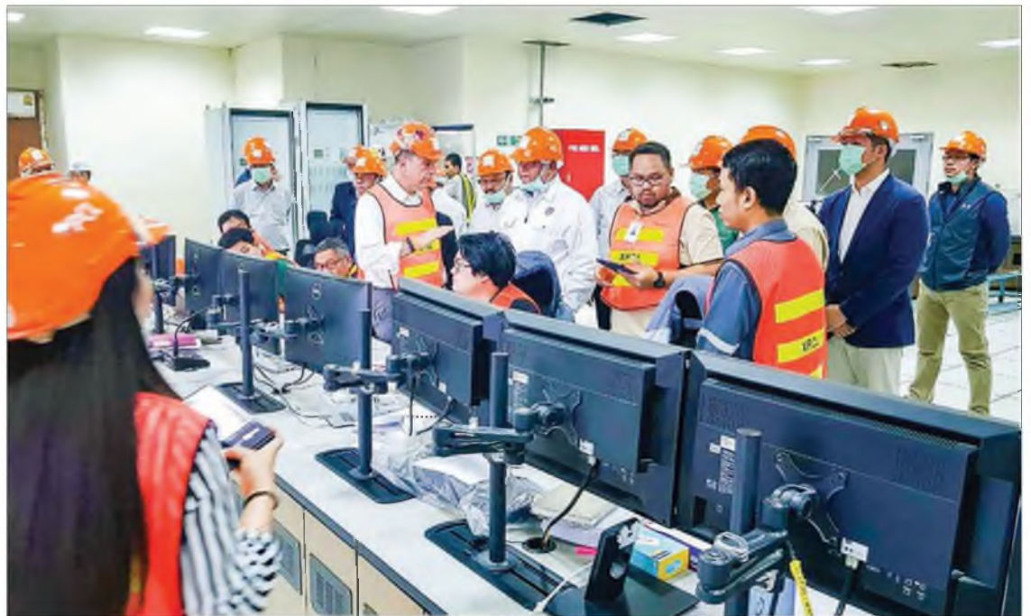
Union Minister U Win Khaing visits the electrical power station in Laos. PHOTO: HTAN PHONE
