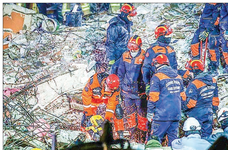
Officials carry out search and rescue missions on the debris of an 8-storey building after it collapsed in Istanbul on 7 February, 2019. PHOTO: KYODO NEWS
