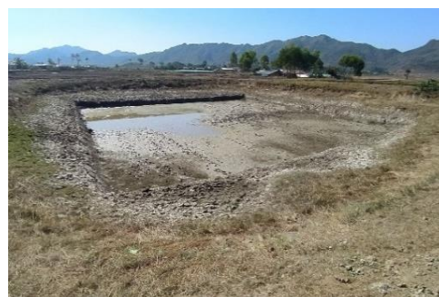
Photo 4 - Pond in KNP before digging and compaction (Feb 23)
