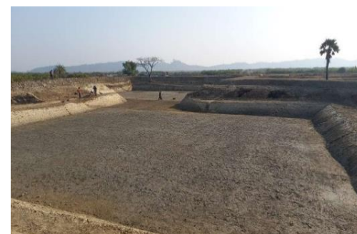
Photo 5 - Pond in KNP after removing dikes, digging and compaction (Mar 23)
