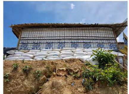
Type 2: Bamboo fencing and tarpuline, plinth level reinforced with sand bags
