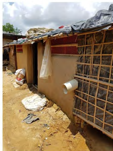
Type 7: Mud and bamboo fencing wall, bamboo and tarpuline for roof
