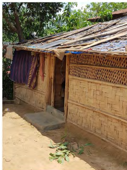
Type 3: Bamboo mesh for wall, tarpuline roof
