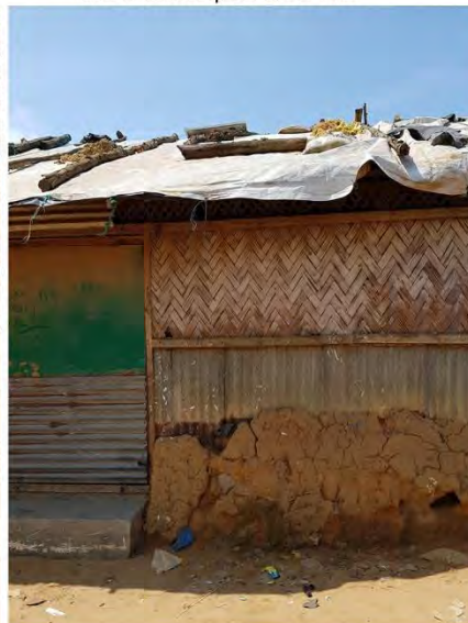
Type 4: Tin and bamboo mesh for wall, straw and tarpuline for roof
