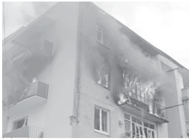
A burning apartment building, damaged by a Russian airstrike is seen the northern Georgian town of Gori.—INTERNET
