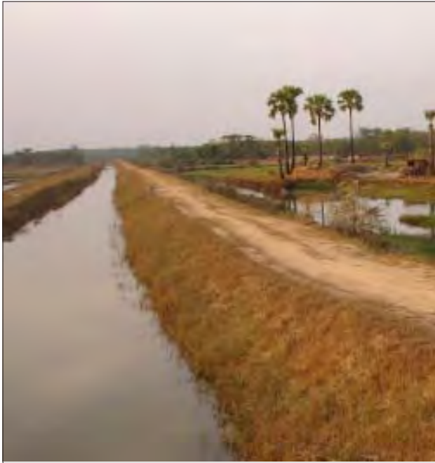
An irrigation cannel from Win-pha-non Dam, Mudon Township
