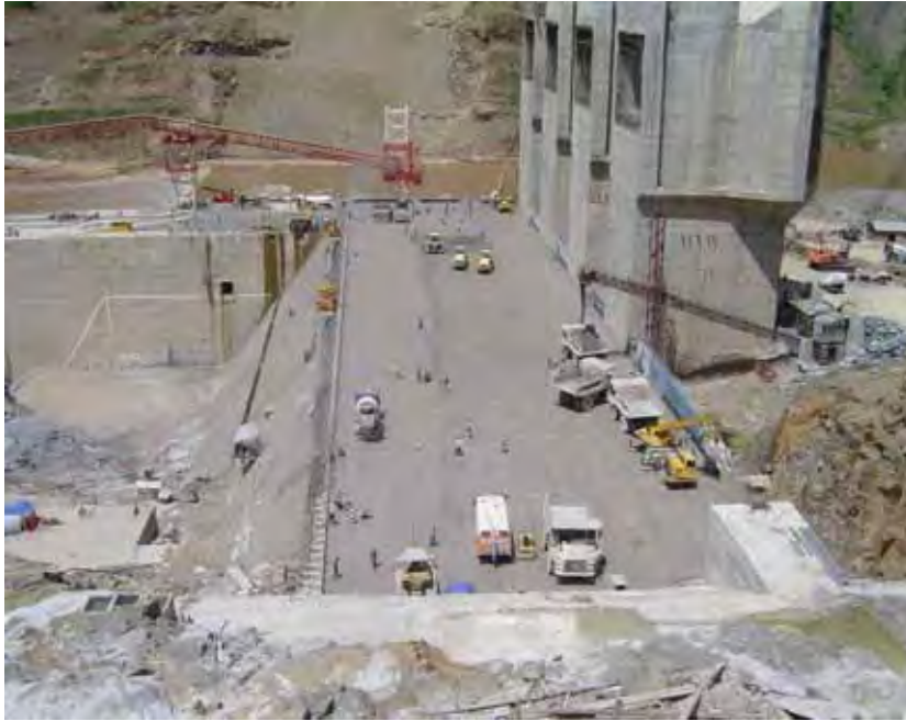
RCC Placing Stage 4a
