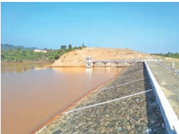
The State government has spared no effort to take measures against bank erosion and to build retaining walls. PHOTO: MNA
