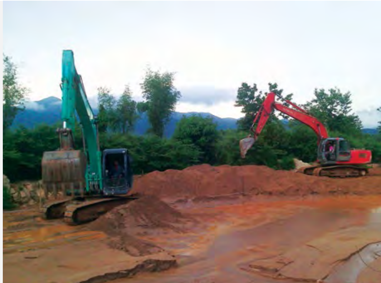
Dredging the Nam Kham stream
