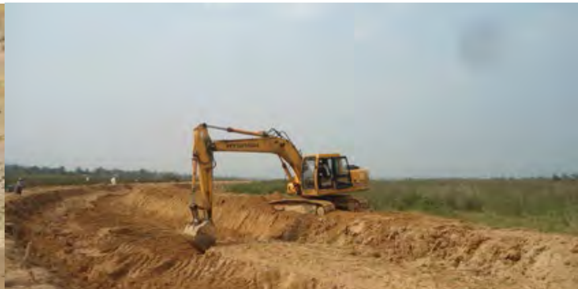
Dredging the Nam Kham stream
