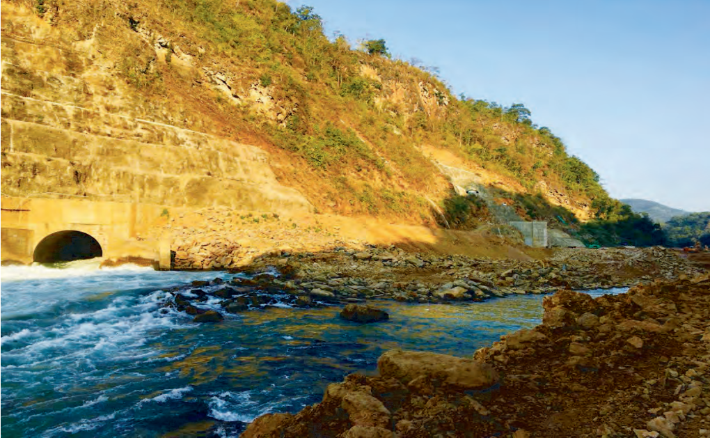
Upper Yeywa dam construction site
