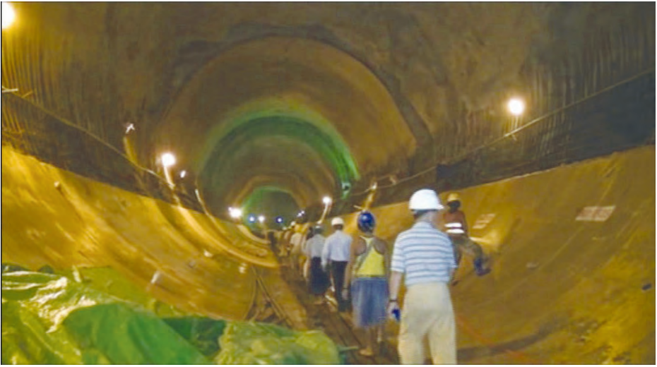
Water diversion tunnel of Upper Yeywa dam
