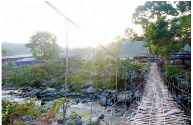
The way across: A wooden bridge links a camp to China
