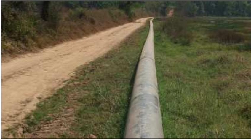
**Pipeline which has not yet been placed in the ground. The ground will be excavated adjacent to the pipeline, dug five feet deep and the pipeline will be placed there.**
