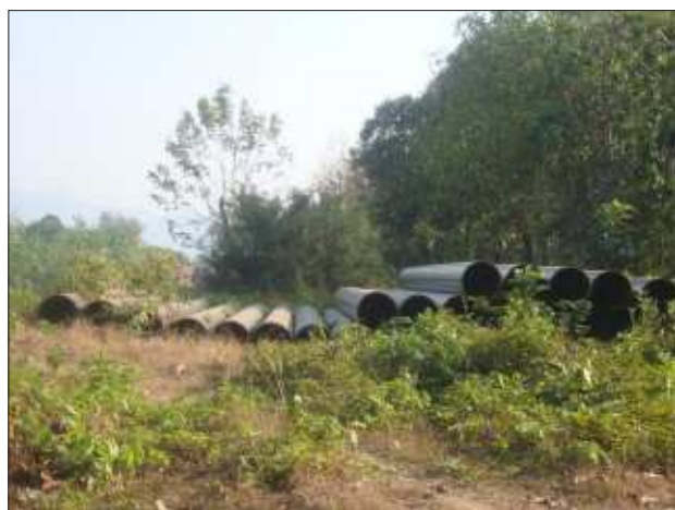
New segments of pipe for the Kanbauk to Myaing Kalay gas pipeline are seen sitting in a pile near Weakhami village, Thanbyuzayat Township.
