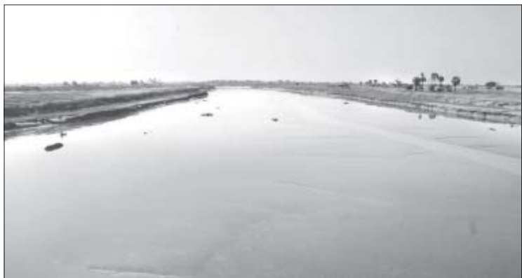
One of the main canals of Kataik dam during the flooding in August in Paung Township
