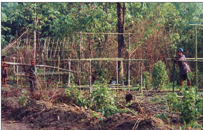
Refugee villagers build huts near Tor Lwi IDPs village.
